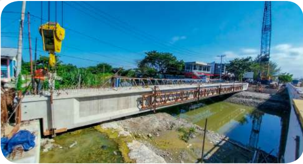
● PCI Girder Krueng Bridge Tukai - Aceh Province
