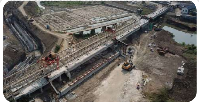
● PCI Girder Glapan Timur Rehabilitation
