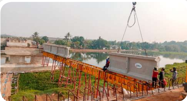
● PCI Girder Walahar Bridge - Karawang
