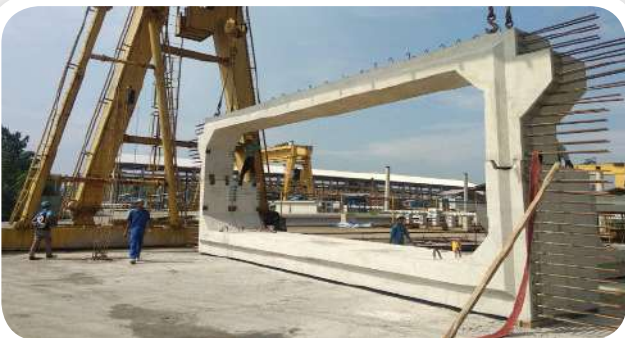
● Box Culvert Grenyang Bojonegoro Bridge
