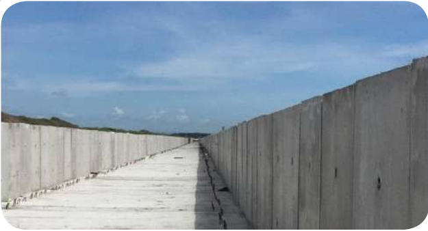
● U-Ditch New Yogyakarta International Airport
