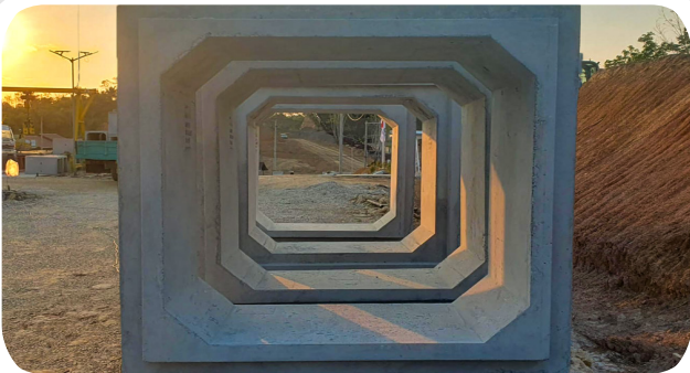
● Box Culvert Feeder Street IKN - East Kalimantan
