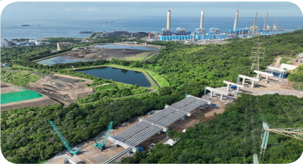
● PCI Girder Probolinggo Banyuwangi Toll Road
