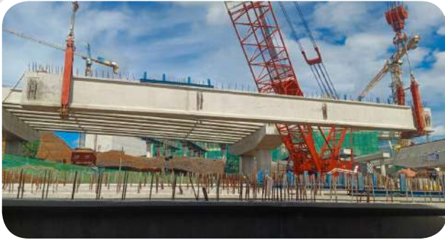
● PCI Girder The Elevated Street President's Office IKN - East Kalimantan
