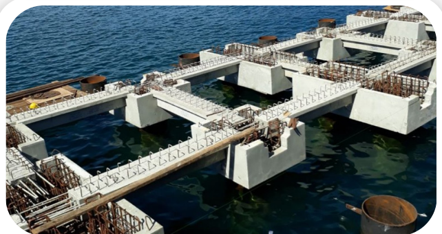
● Jetty Construction Piabung Port
