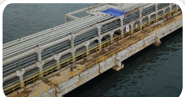
● Pipe Rack Tanjung Batu Balikpapan Jetty
