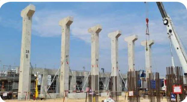
● Pipe Rack Freeport Smelter Gresik
