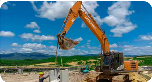
● U-Ditch Feeder Street IKN - East Kalimantan
