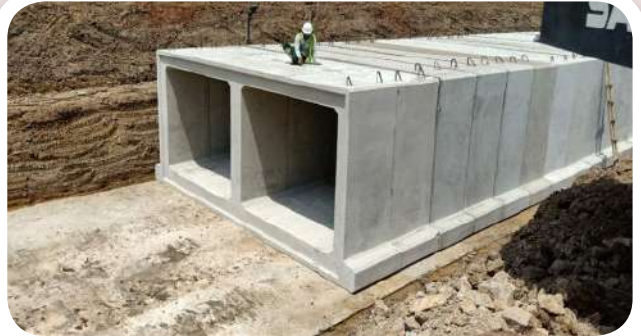
● Box Culvert New Yogyakarta International Airport
