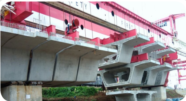
● Box Girder Double Double Track Manggarai
