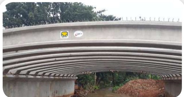
● Curved PCI Girder UIII Campus Main Gate Bridge Depok
