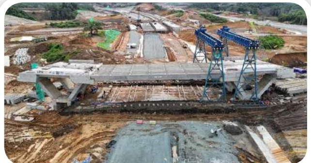
● PCI Girder VVIP Airport IKN - East Kalimantan
