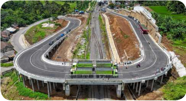
● Spun Pile, Square Pile, PCI Girder, Diaphragm Precast Bridge Maseng, Bogor, West Java
