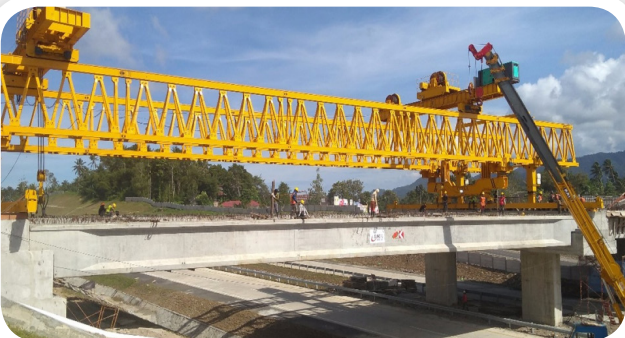
● PCI Girder Manado Bitung Toll Road
