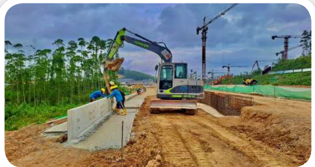
● L-Shape Sumbu Barat Street IKN - East Kalimantan
