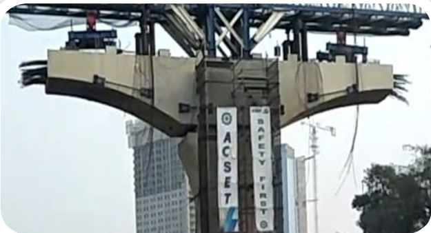
● Pier Head Precast Jakarta - Cikampek 2 Elevated Toll Road
