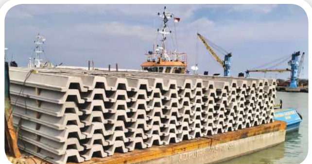
● Corugated Concrete Sheet Pile (CCSP) Veteran River Banjarmasin City Phase 1 - South Kalimantan
