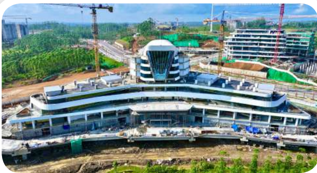
● PCI Girder Bank Indonesia IKN - East Kalimantan
