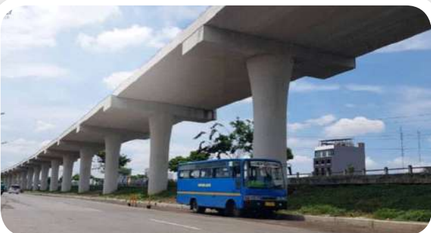
● Voided Slab JLNT Pluit By Pass
