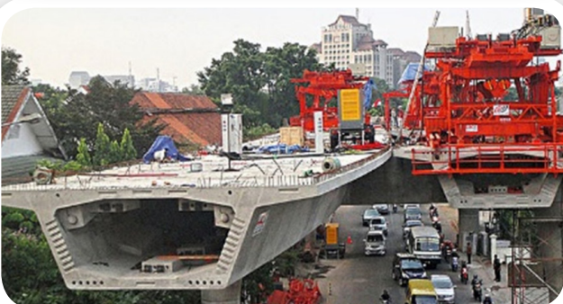
● Box Girder Bogor Outer Ring Road
