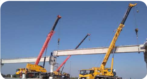
● PCI Girder Solo-Kertosono (SOKER) Toll Road - Central Java
