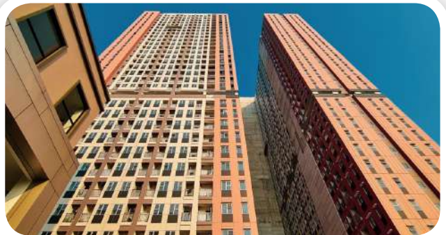
● Facade Transpark Mall Juanda - Bekasi
