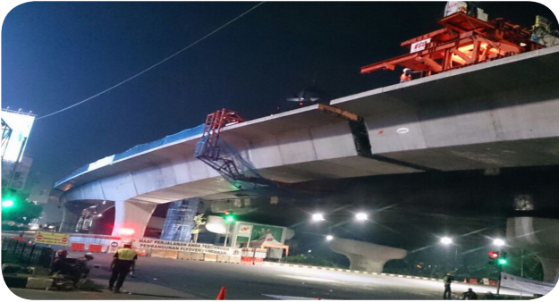
● Box Girder Pancoran Fly Over
