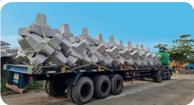
● A-Jack Toll Road Development Semarang - Demak
