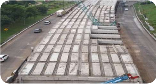
● Full Slab Boulevard Deltamas Fly Over
