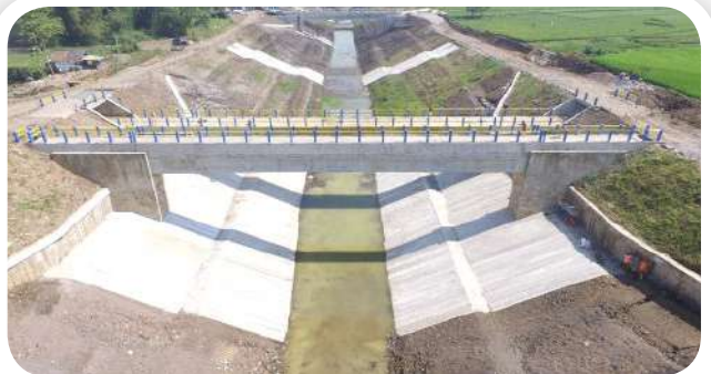
● Lining Cisangkuy Irrigation
