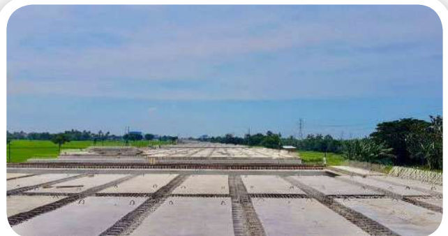
● Full Slab Cibitung Cilincing Toll
