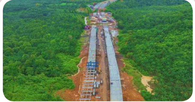
● Full Slab, Half Slab Outer Ring Road IKN - East Kalimantan
