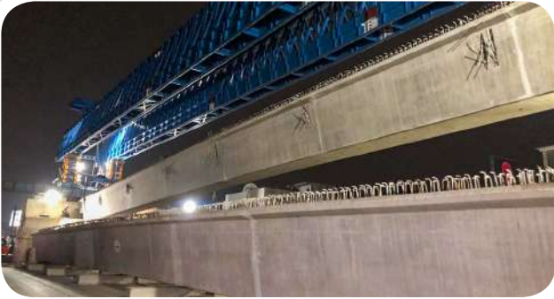
● PCI Girder Cisauk Bridge Tangerang - Banten
