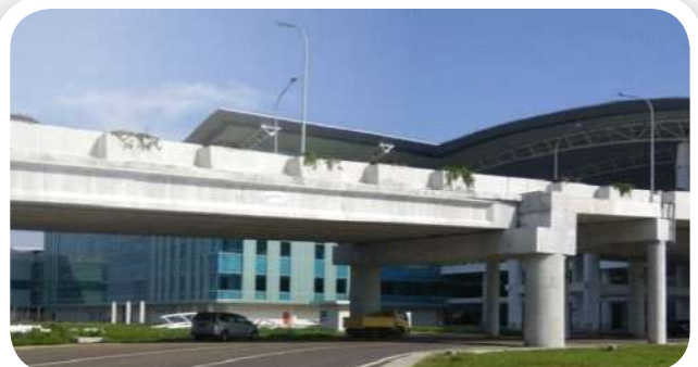
● Voided Slab Entrance Access Kertajati Airport
