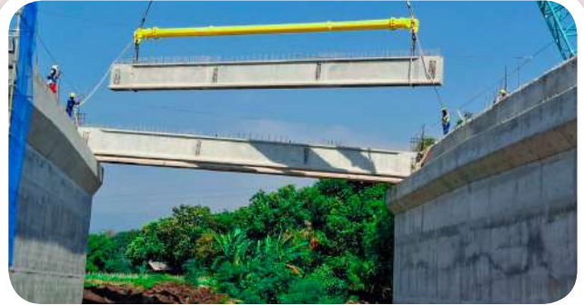
● PCI Girder Probowangi - East Java
