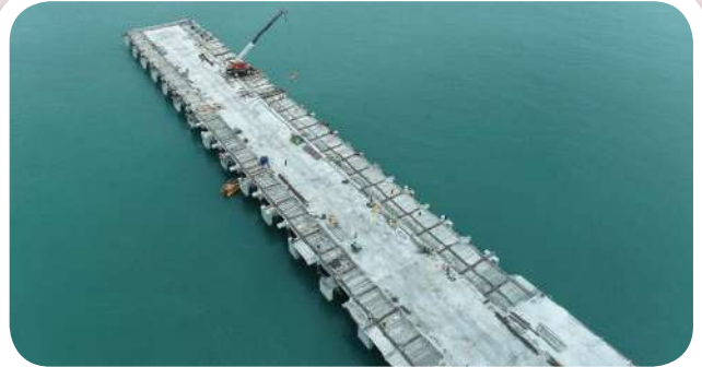
● Jetty Construction Tuban Port, East Java
