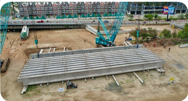
● PCI Girder C-D Island Connection Bridge Pantai Indah Kapuk 2
